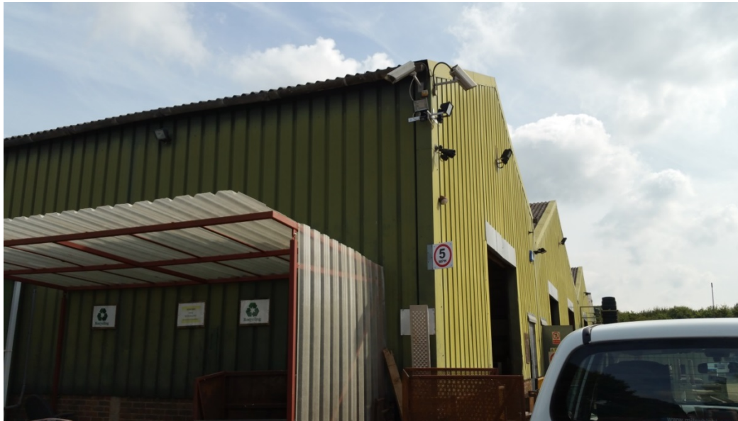
Figure 3: Existing lights on Units 1 to 3
